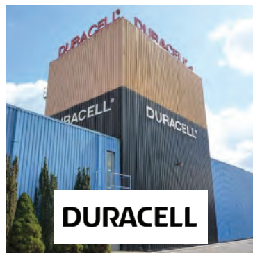
Duracell Batteries Belgium
